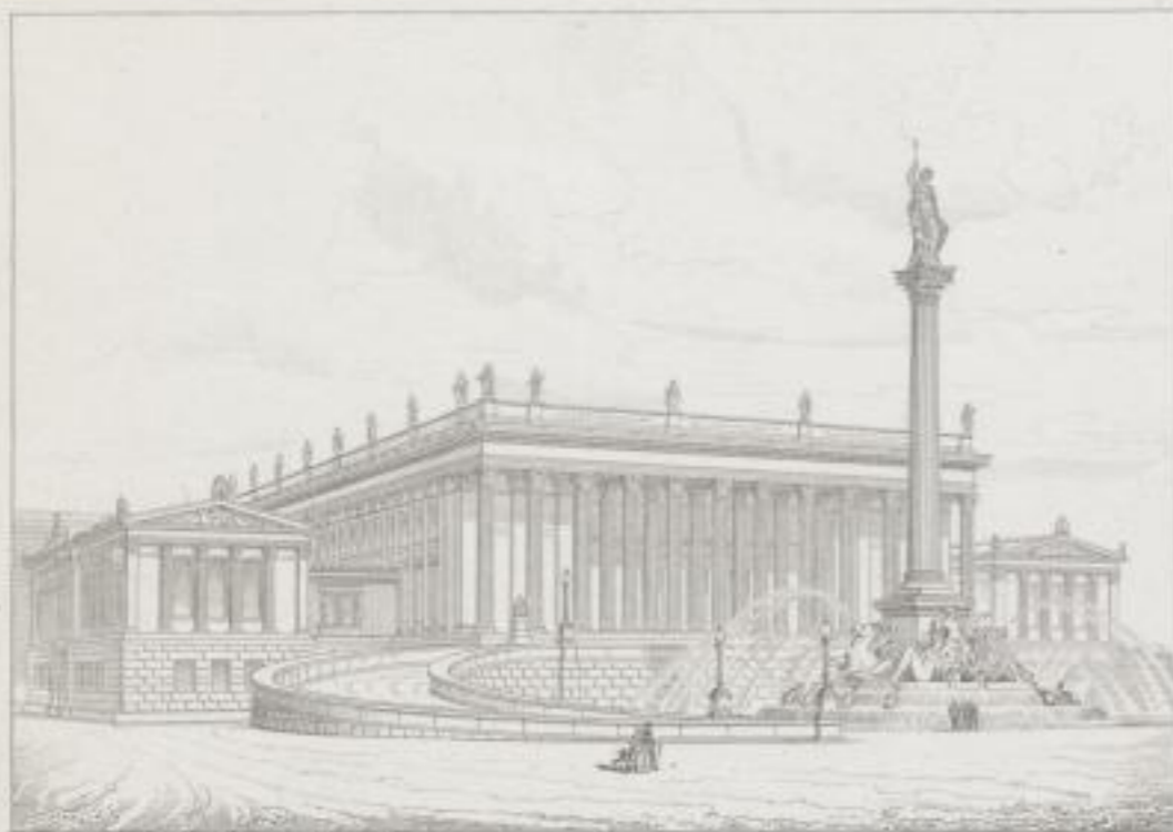
Facade des Herrenhauses in Wien (Sanson)
