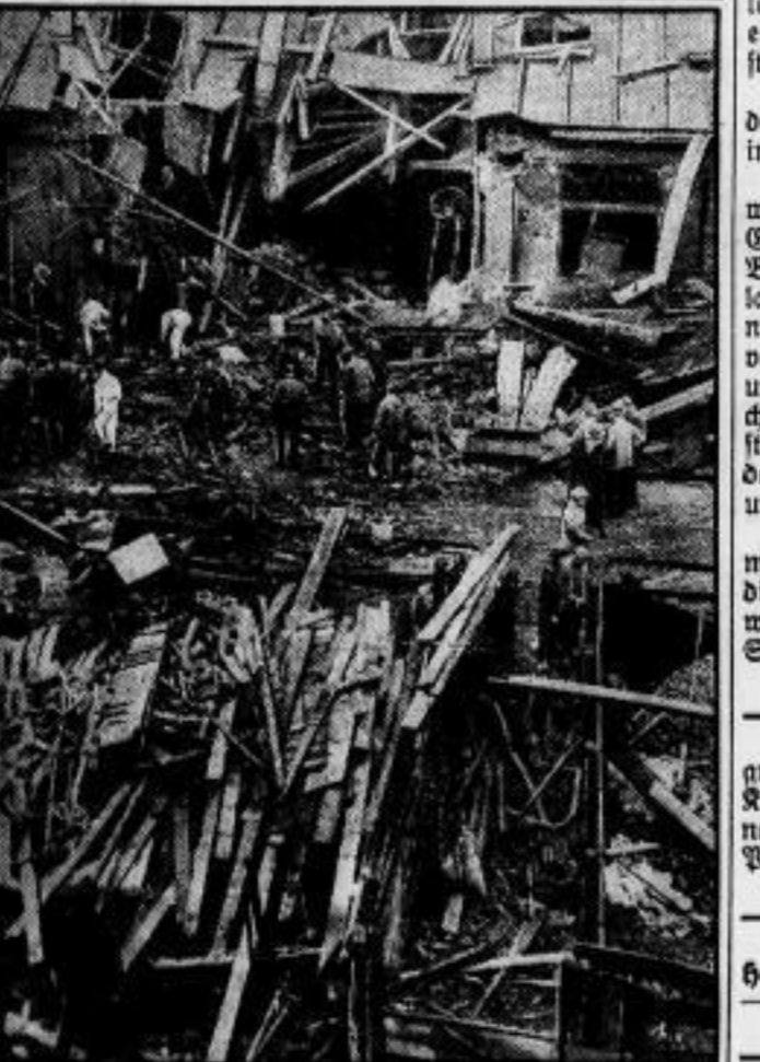
Schwere Explosion in Utrecht.
