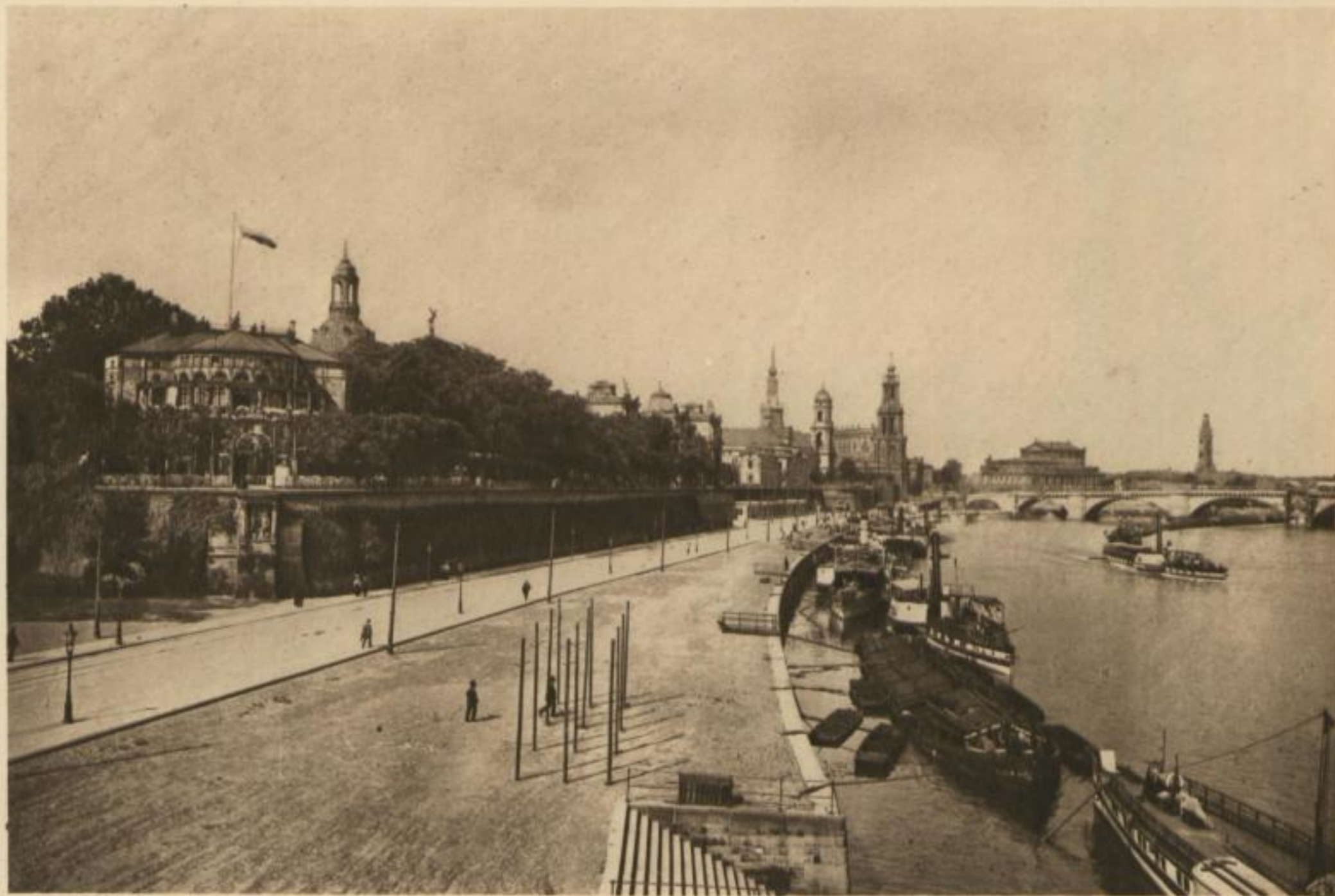
- View from the Queen Carola-Bridge.
