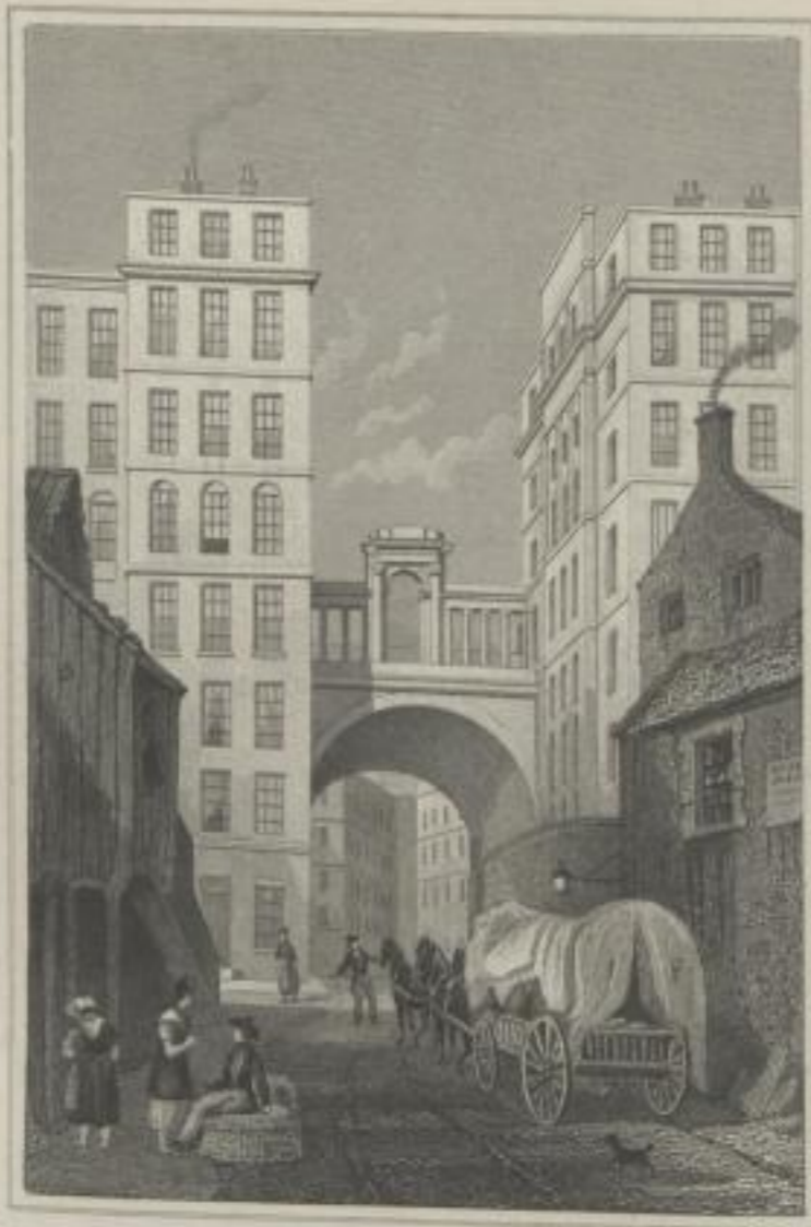
THE REGENT BRIDGE.
