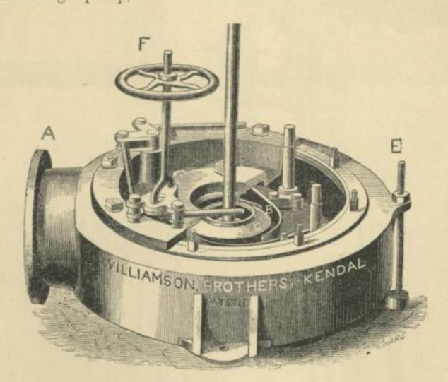
PATENT VORTEX TURBINE, an improved means of applying water-power.
